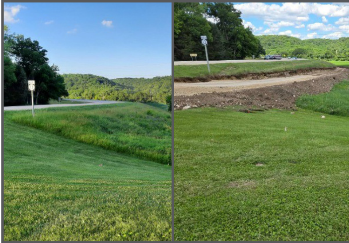
Pony Hollow Trail: Before and During Construction
